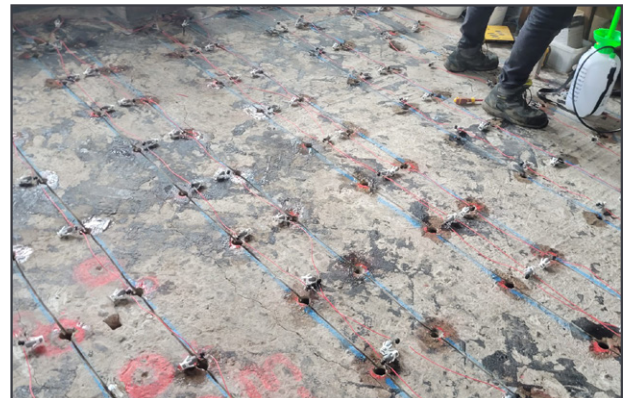
DuoGuard™ installation in floors
