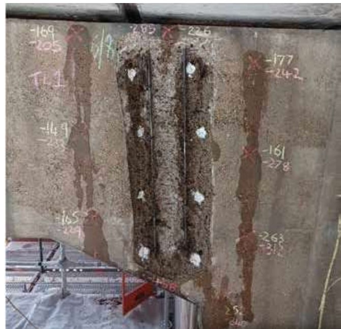
Figure 3: Steel Potentials were Recorded Before (Yellow) and After (Pink) Connection of The Galvanic Anodes.
