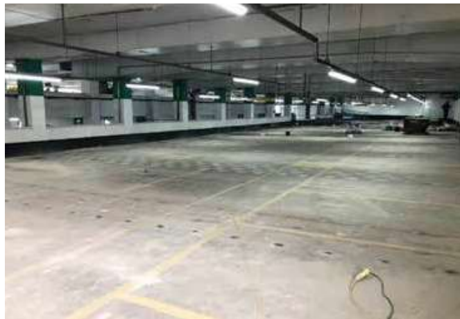
Figure 11: Car Park Deck Photo Taken After Installation of Anodes Before the Application of Deck Coatings.
