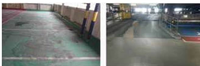
Figure 8: Evidence of Poor Drainage (Left), Membrane Wear (Right) Observed in 2023.
