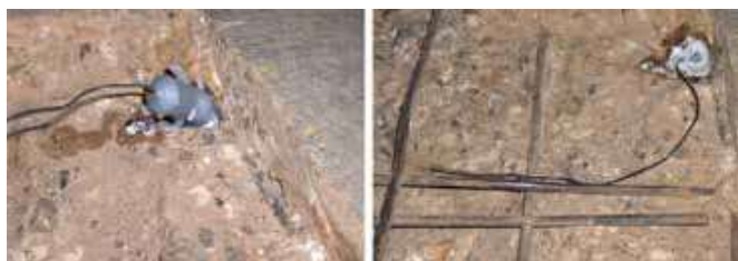
Figure 5: Installation of Anode in Parent Concrete at Repair Edge and its Connection to the Steel in 2010.
