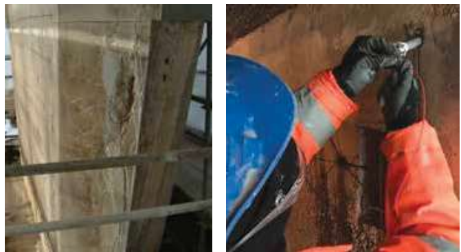
Figure 13. Example of the Damage (Left) and Repair Using Anodes (Right) on the Bridge Piers in 2007.
