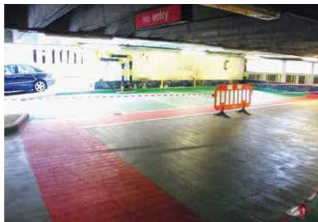
Figure 7: Coating or Membrane Applied to the Decks of The Grosvenor Car Park in 2011.
