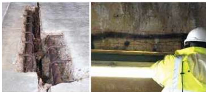
Figure 4: Examples of Corrosion Damage Observed During the Repair of the Car Park in 2010 and 2011.
