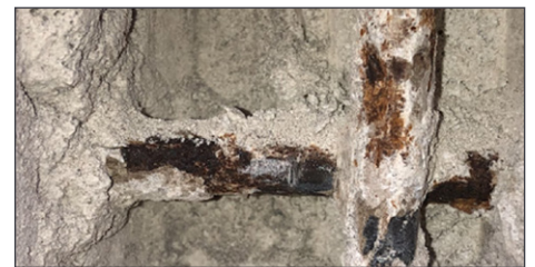
Example of corrosion in RAAC
