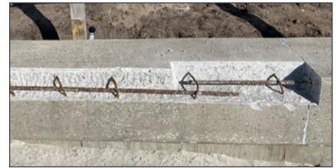
Sea wall cap reinforcement
