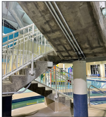
PatchGuard Connect HiFlow installation
