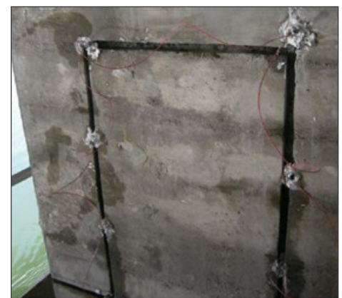
DuoGuard installation prior to infilling holes and saw cuts
