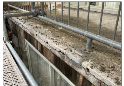
Close up of balcony edge showing position of installed anodes
