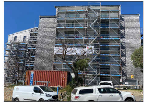
Twin Towers Building works on site
