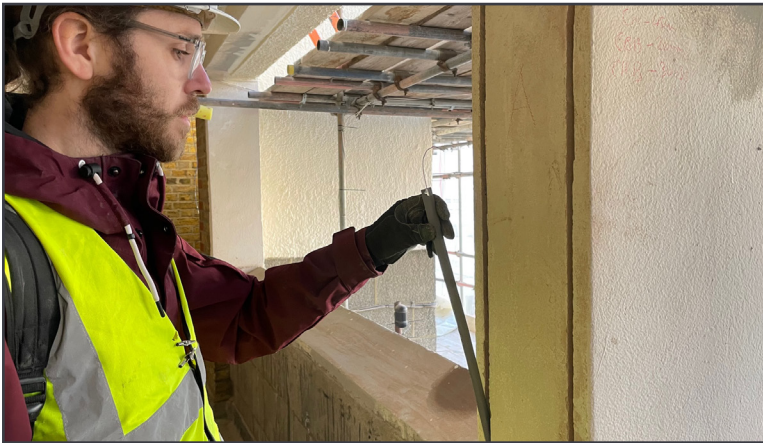
PatchGuard Strip placement in sawcuts
