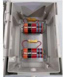
A lockable cabinet which facilitates performance monitoring measurements of CPT corrosion protection systems
