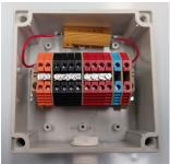
A connection box which facilitates performance monitoring measurements of CPT corrosion protection systems
