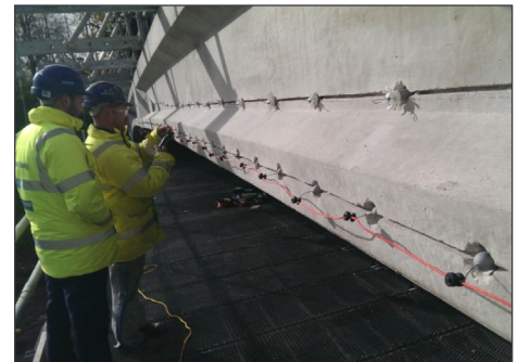
Sherbourne Bridge anode installation
