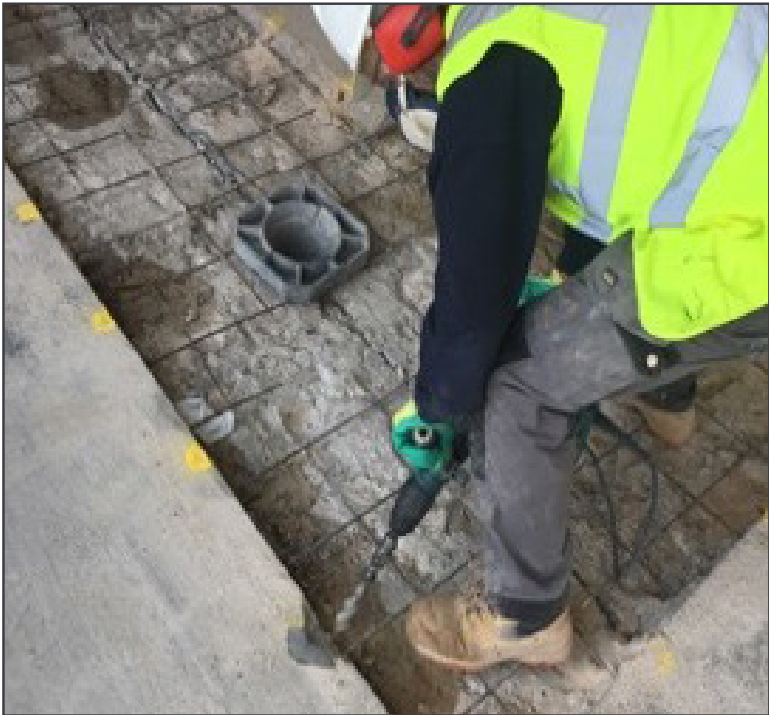
Installation of anodes
