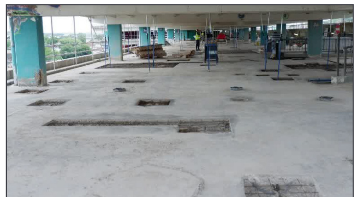
Breakout of the car park decks
