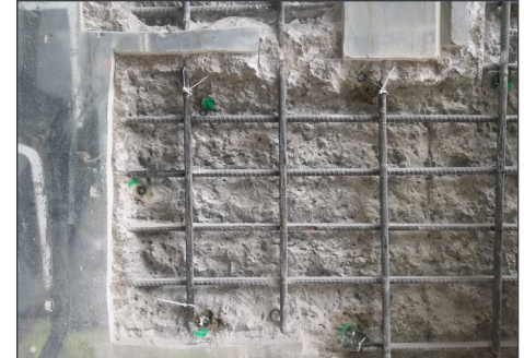
Anodes to perimeter of repair
