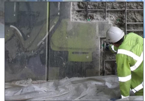
Type 1b anodes being installed to abutment repair
