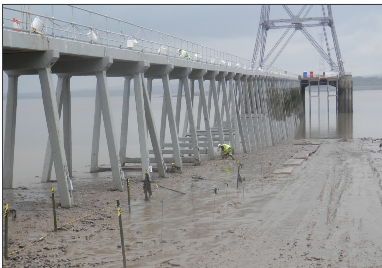
Bulk anodes in tidal zone.
