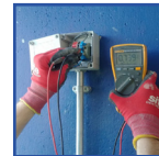
CPT Monitoring System
