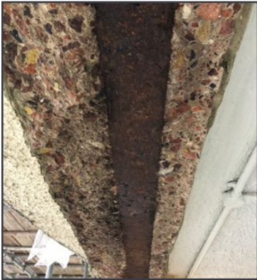
Corrosion of beam flange
