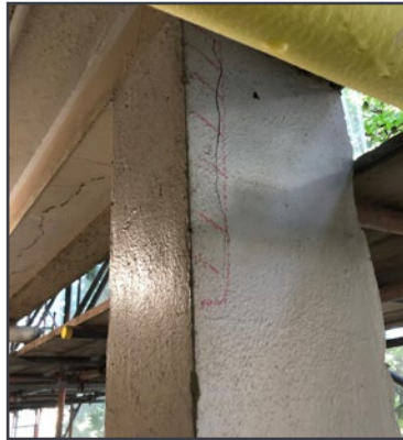
Cracking and delamination
