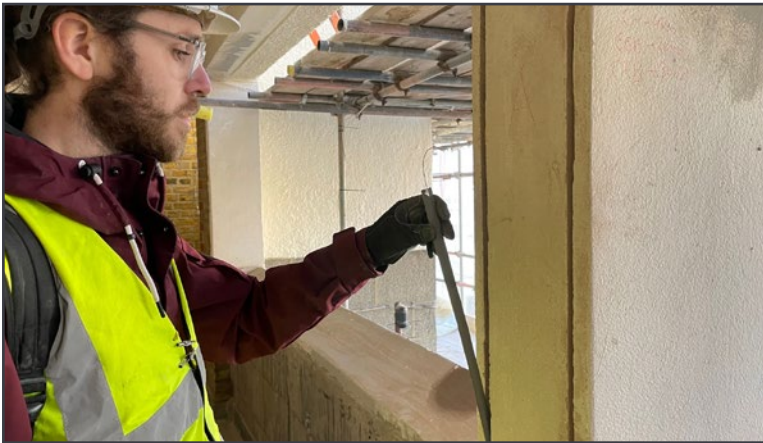
PatchGuard Strip placement in sawcuts
