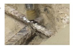
**3.** Check the resistivity of the multimeter and cables prior to use by touching the pins together as shown. Subtract this value from subsequent measurements to give a true resistivity reading. Confirm steel reinforcement continuity in areas to be treated by checking a sample of bars within the patch.
