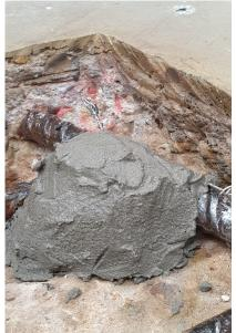
NOTE: Insulating patch repair materials and primers (eg. Epoxy modified) shall not be used with the RebaGuard anodes as this compromise current flow from the anodes to the parent concrete outside the patch.
