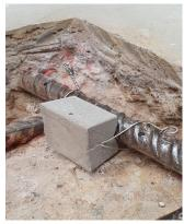
Use a multimeter to measure the resistance between the (clean) steel bar and the wire protruding from the RebaGuard unit. Resistance must be **less than 0.50 ohm,** if not, then the anode must be removed and re-attached.
