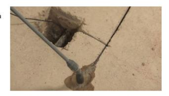
**6.** Strip the coating from the titanium wire using wire strippers, only in the location where the anodes are to be fixed. With the PatchGuard Connect anodes positioned in the holes electrically connect the individual units to the titanium feeder wire using the plastic screw connector.
