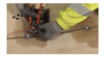
Tighten with a 12mm (½") ring spanner ring spanner. Twist the excess wire from the PatchGuard Connect units around the titanium feeder wire to ensure electrical continuity.
