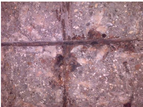
**Fig. 5.** Chloride pitting on the steel broken out during the repair of H6 canal bridge
