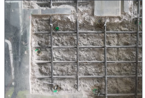
Anodes to perimeter of repair
