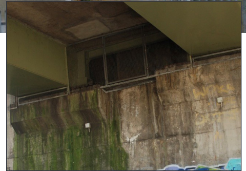
View of abutment
