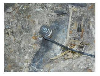
**8.** If monitoring is to be installed, cables from the installed ProtectorJoint anodes, steel and reference electrodes should be joined to multi-core cable using a cable joint kit prior to running to the monitoring enclosure (optional).
