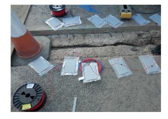
7. Make connections to the steel reinforcement at locations identified in the design or as agreed with the engineer. The type of steel connection used will be dependant on the electrical conductor utilised for the negative connection. Measure the current flowing between the steel and the anode string to confirm operation of the system.
