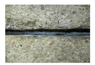
**10.** Connect the string of ProtectorJoint anodes either directly to the steel reinforcement or into the monitoring enclosure.
