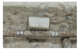
Use a multimeter to measure the resistance between the (clean) steel bar and the wire protruding from the RebaGuard unit. Resistance must be **less than 0.50 ohm,** if not, then the anode must be removed and re-attached.
