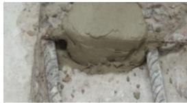
**8**. Patch repair material cover to the RebaGuard unit must be a minimum of 20mm. The patch repair should be completed ensuring the RebaGuard unit is not disturbed.
