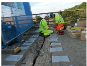
**3.** If units incorporating reference electrodes are used these should be installed within the string of ProtectorJoint units. Note the blue cable from the reference electrode unit in the photograph.
