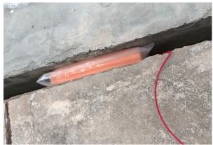
7. Make connections to the steel reinforcement at locations identified in the design or as agreed with the engineer. The type of steel connection used will be dependant on the electrical conductor utilised for the negative connection. Measure the current flowing between the steel and the anode string to confirm operation of the system.
