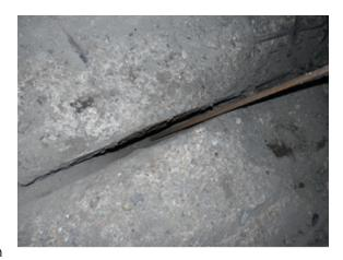
**2.** Pre-connect the ProtectorJoint anode units to the titanium feeder wire at the design spacing and securely tighten screw connectors using a ring spanner. Twist excess wire from each unit around feeder wire, as shown, to ensure electrical continuity. Measure the electrical resistance between the titanium feeder wire and the individual ProtectorJoint anode units following connection. The resistance shall be less than 0.5 ohm.
