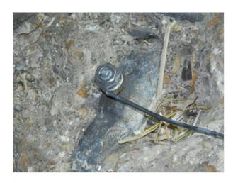
**8.** If monitoring is to be installed, cables from the installed ProtectorJoint anodes, steel and reference electrodes should be joined to multi-core cable using a cable joint kit prior to running to the monitoring enclosure (optional).
