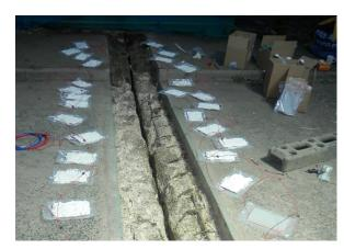
**5.** The individual anode units are placed into the joint and inserted such that the face of the unit coated in embedment material is in contact with the concrete joint face. The anode units are located such that a gap of 20mm is present between the top of the anode unit and the joint fill material. The titanium feeder wire will be located within the joint below the proposed location of fill material.
