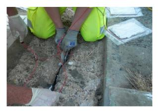
**6.** Puncture the plastic enclosure to allow the compressed foam to expand and fill the joint gap.
