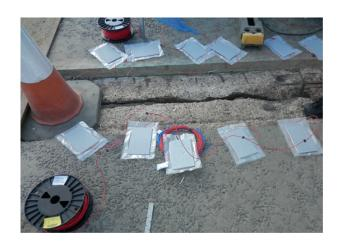
**4.** Coat the ProtectorJoint anode surface with the DuoCrete J activating adhesive, using a spatula or roller. Do not leave the coated anode units exposed for greater than 30 minutes to avoid drying of the embedment material.
