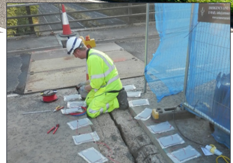
Onsite installation of ProtectorJoint™
