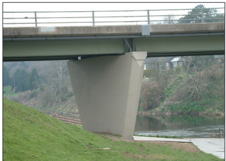
Finished pier 10 years after installation
