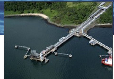
Braefoot Jetty Aerial View
