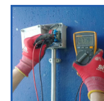
CPT Monitoring System
