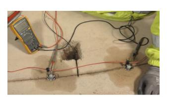
7. Remove the PatchGuard Connect anodes from the holes. Using a caulking gun and a rubber hose extension apply DuoCrete PG mortar, ensuring that any trapped air is removed. Fill the pre-drilled holes approximately half way up with the mortar. Insert the individual PatchGuard Connect units into the mortar. The mortar should flow to ~20mm (1/8") from the concrete surface. The plastic screw connector must be 20mm (1/8") below the concrete surface.
