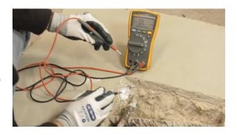
Repeat this process until a resistance of 0.5 ohm or less is achieved then secure the anode wire to the steel using 2 plastic cable ties.
