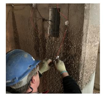
**11.** Check the installation for electrical shorts by measuring the electrical potential between the reinforcing steel and the DuoGuard units using a high impedance voltmeter during installation. The potential difference should be greater than 300 mV and stable.
