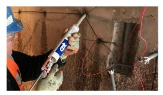
**10.** Insert the DuoGuard units into the mortar. The mortar should flow to ~20mm (7/8") from the concrete surface. The plastic screw connector must be 20mm (7/8") below the concrete surface.
