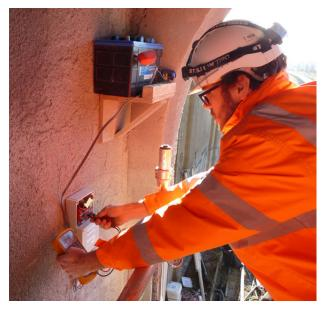
14. Activate the power supply within 2 hours of installation of the DuoGuard anode units.
