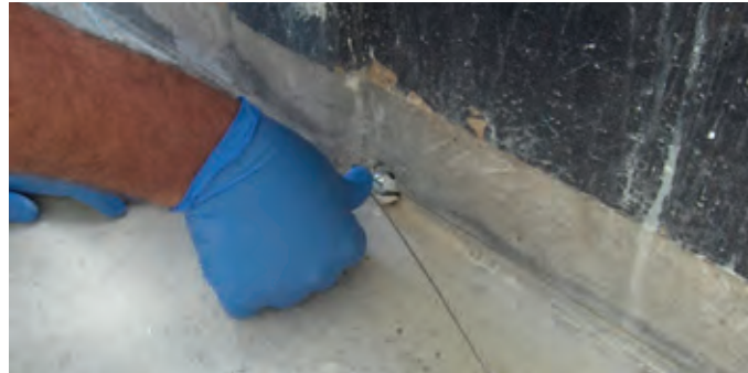
◀ ▶ DuoGuard [hybrid] anode installation
