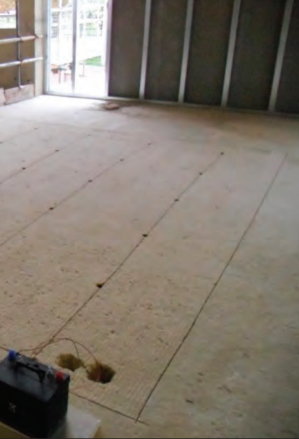
◀ ▶ DuoGuard [hybrid] anode installation
