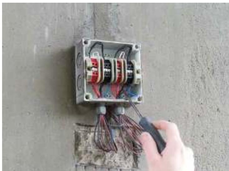
Figure 40 - Arrangement of terminal block connections
