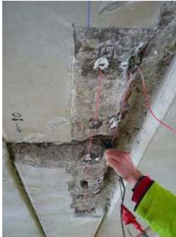
Figure 5 - Installation of Hybrid anode system in pre-stressed concrete beams
