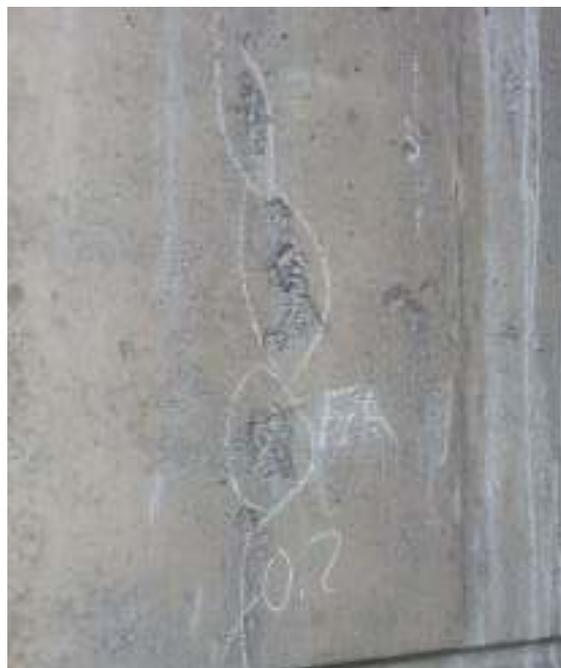
Figure 43 - Surface defects (honeycombing) to abutment at Junction 2
