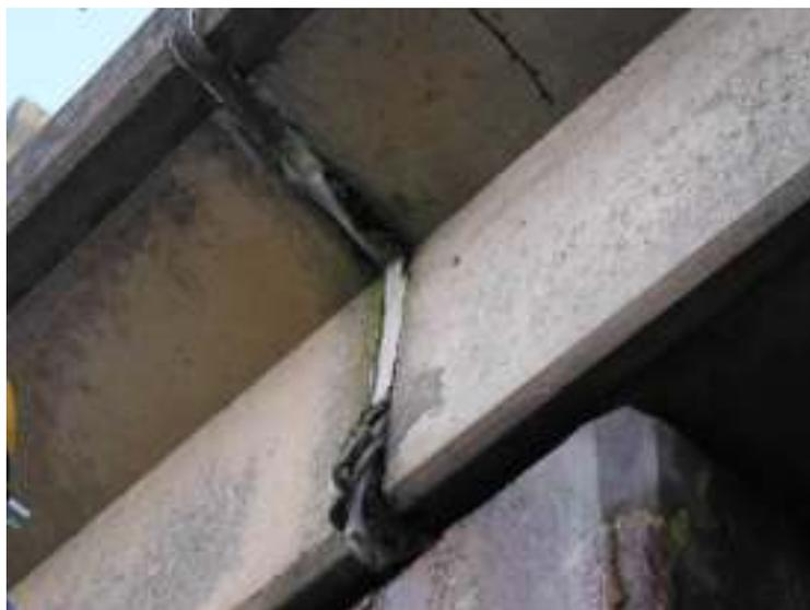
Figure 34 - Deterioration of bridge joints above abutment walls
