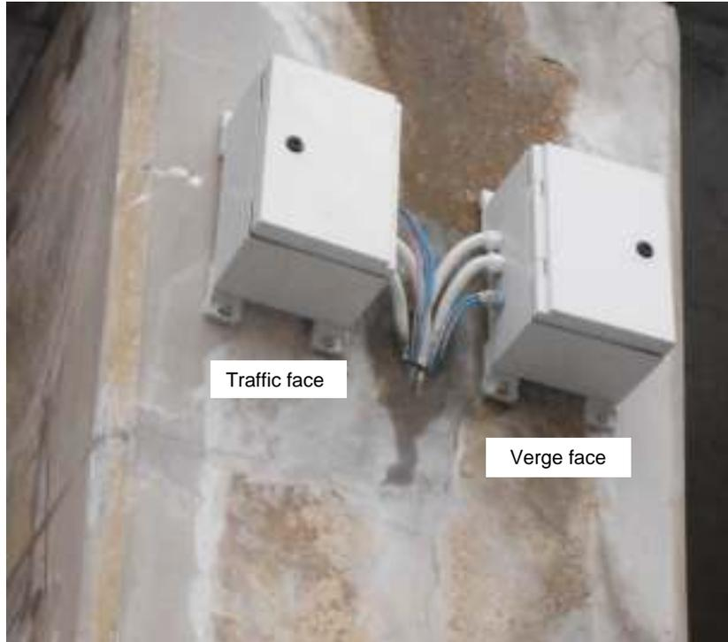
Figure 30 - Junction boxes located on the end of abutments
