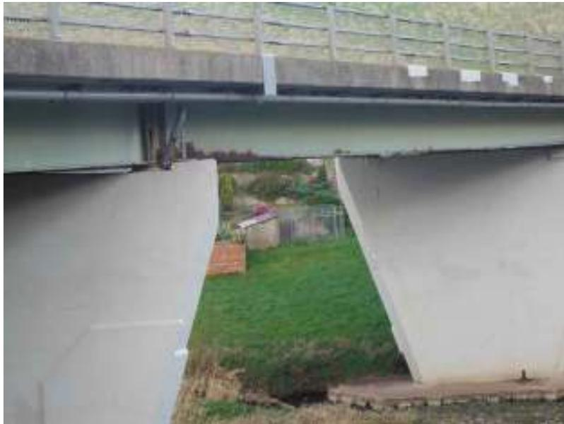
Figure 12 - Corrosion of steel girders in close proximity of bridge joints
