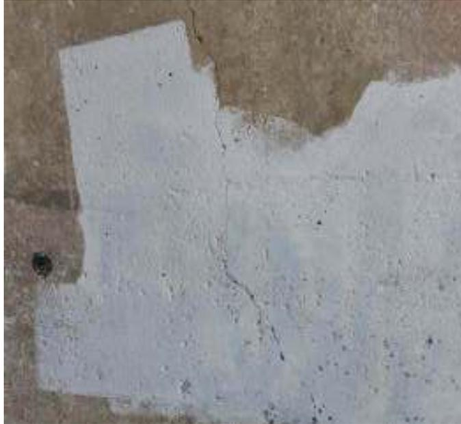
Figure 25 - Shrinkage cracking to North abutment
