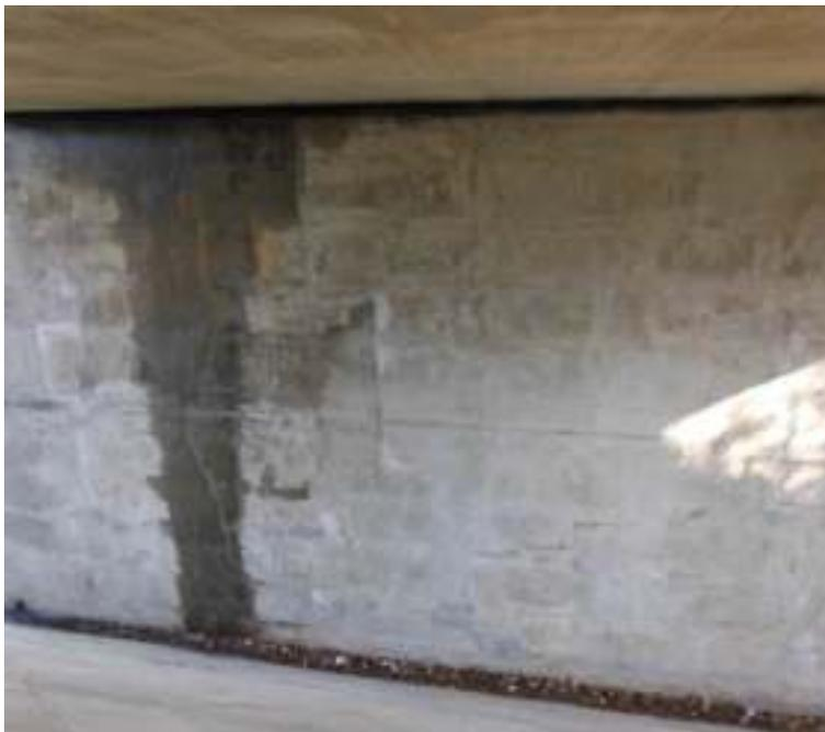
Figure 35 - Evidence of water ingress (North-West abutment, verge face)
