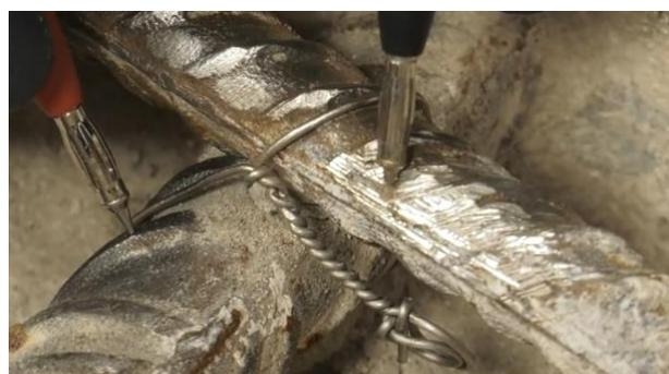
4. Drill 25mm (1") holes of the required depth at the edge of the patch repair (see table) making sure to avoid contact with the steel. Remove excess dust.
