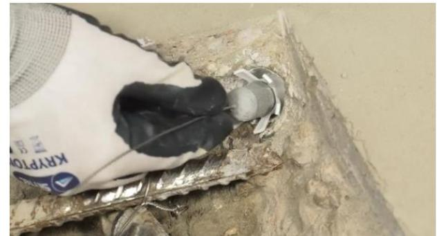
**7. Connect the PatchGuard by wrapping the anode tying wire (minimum 2 times) around the pre-cleaned steel bar and carefully tightening using pliers.**
