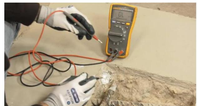
Repeat this process until a resistance of 0.5 ohm or less is achieved then secure the anode wire to the steel using 2 plastic cable ties.
