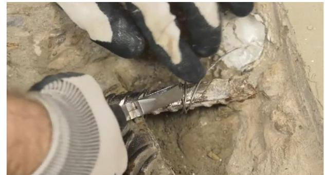
**8. The electrical resistance between the connecting wire on the PatchGuard anode and the reinforcing steel should be confirmed to be 0.5 ohm or less.**
