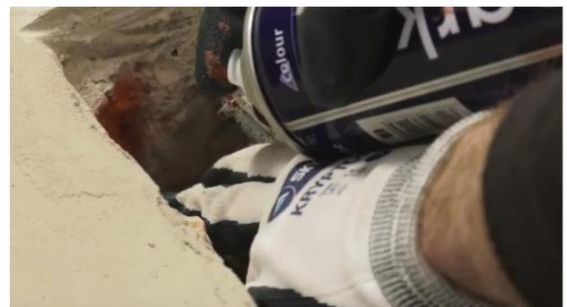
**2.** Clean the steel, using a wire brush or file, in the vicinity of the proposed location of the PatchGuard anode to facilitate electrical connection.
