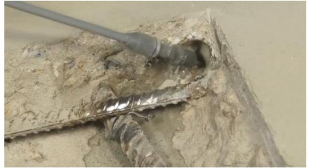
**6. Insert DuoGuard PG cartridge into caulking gun. Cut off the end of the nozzle with a sharp knife and squeeze trigger, 1 or 2 pulls, to expel any watery material before proceeding.**
