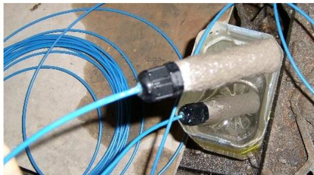
**7. Remove dust and debris and then, using a spray bottle or other suitable method, wet out the anode holes for a **minimum of 15 minutes** ensuring that any excess water is removed prior to application of the SD mortar.**
