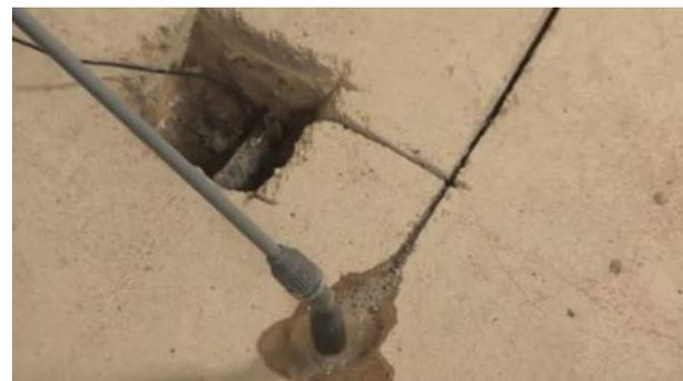
**8.** Using wire strippers, strip the coating from the red insulated titanium feeder wire at the locations where the anodes are to be fixed. With the DuoGuard Anodes positioned in the holes electrically connect the individual units to the titanium feeder wire using the plastic screw connectors.
