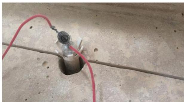
Check the connection between the DuoGuard anodes and the feeder wire by using a multi meter to ensure a resistivity of 0.5 ohm or less.
