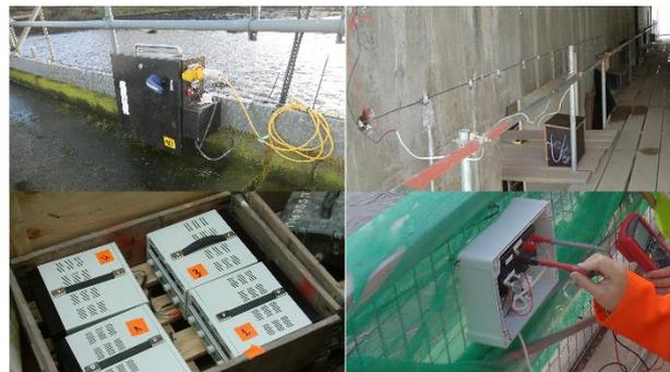
**6. Pre-soak CPT MN15 reference electrodes in saturated lime water and install at marked locations into typically 105mm (4 1/8") deep x 30mm (1 1/4") diameter pre-soaked holes, using a suitable bedding mortar. Run the cabling back in 20mm (7/8") deep x 7mm (1/4") wide saw cuts to the appropriate terminal within the connection box.**
