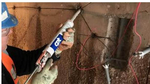
DuoCrete SD mortar should only be applied and cured at a temperature greater than 5°C and rising.
