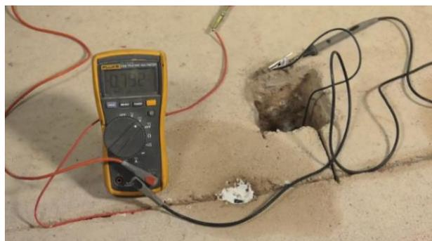
**12.** The remaining void at the top of the anode hole shall be filled with a low shrink repair mortar within **2 hours of installation.**
