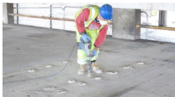
Ensure that no reinforcing steel is exposed within the holes and saw cuts as this has the potential to cause electrical shorts.
