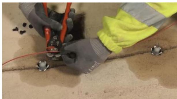
Carefully tighten the connectors with a 12mm ( $\frac{1}{2}$ " multi-tooth ring spanner/socket. Twist the excess wire from the DuoGuard units around the titanium feeder wire (as shown) to ensure electrical continuity.
